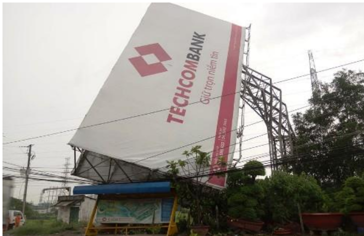
Figure 2. Damage of Billboard (Dong An industrial area, Binh Duong province, 7 August 2013) [6]
