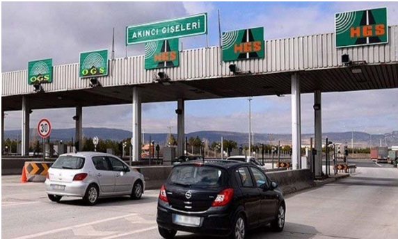
Fig. 6 Ankara highway entrance HGS reading point
