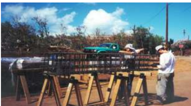
Fig. 5. Off-Site Column Fixing (Future State)
