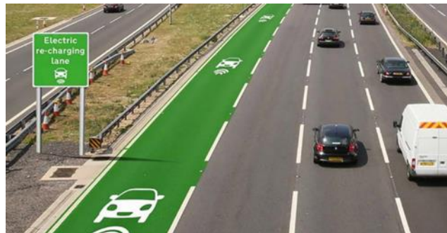
Figure 6: A dynamic charging lane on roadway
